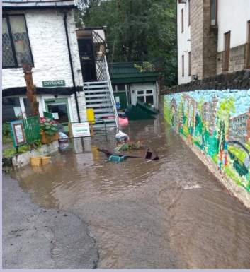
Floodwater pouring in at the front of the Centre
